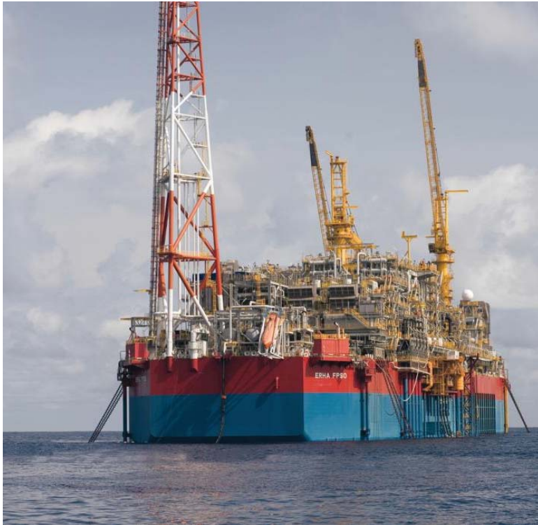
Erha FPSO, offshore Nigeria
